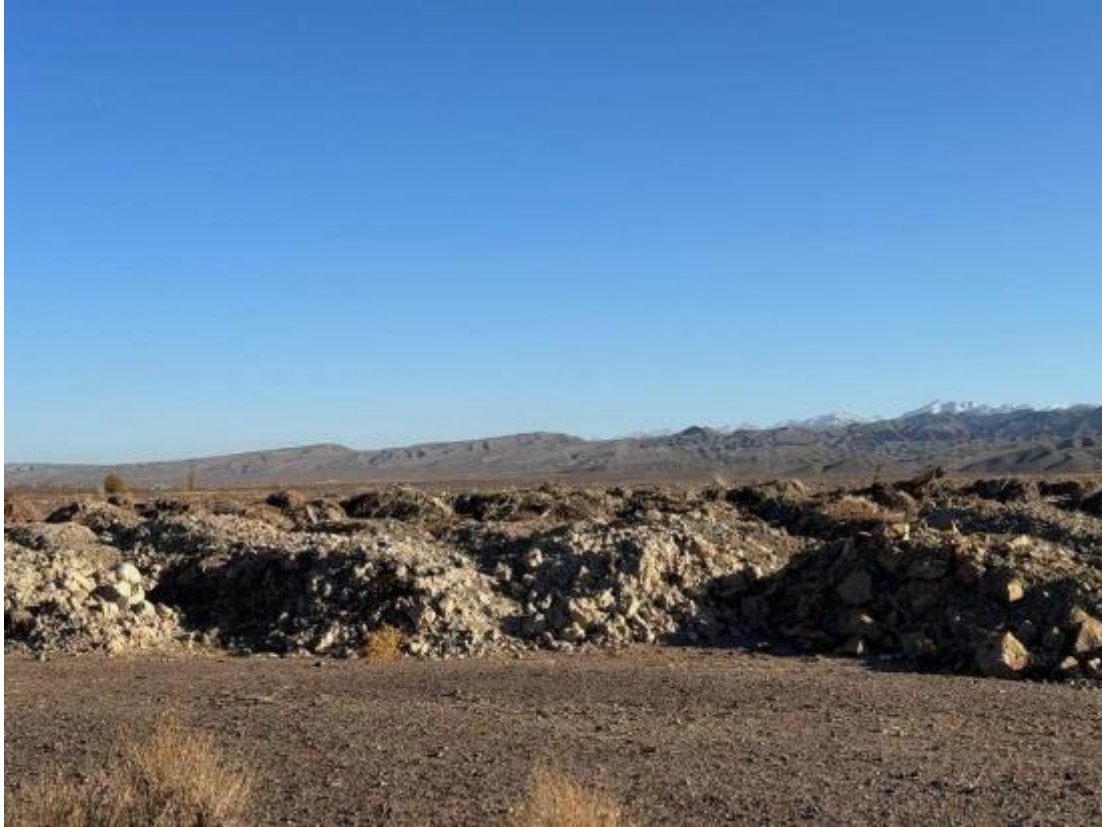
Photo 12. Dumps of construction waste, unsuitable soil/
