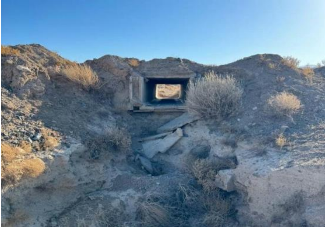
Photo 9. Condition of head/wing of drainage structures at outlet.
