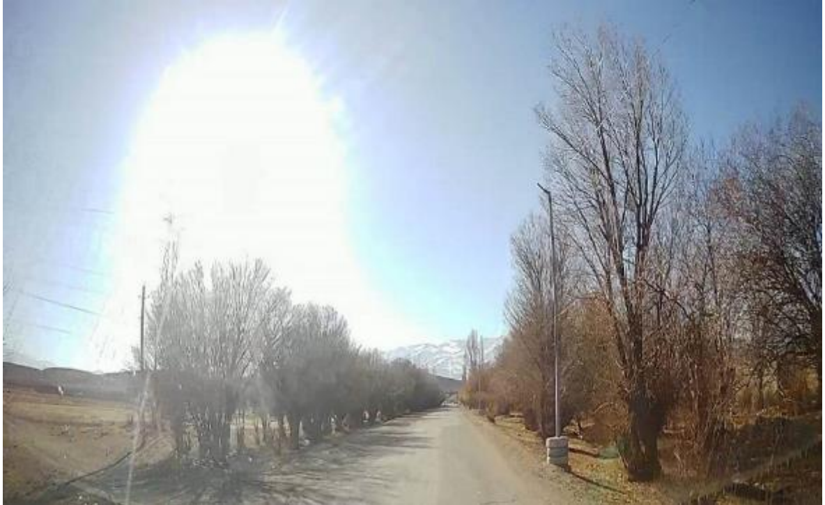
Photo 43. End of section of access road from Kochkor-Epkin highway (chainage 81+400) to Cholpon v.
