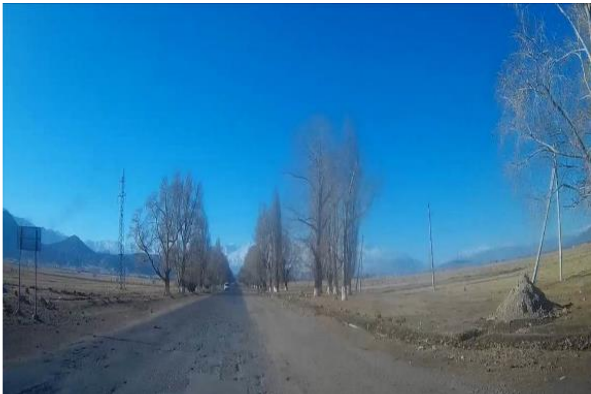
Photo 16. Beginning of Tendik-Roundabout road section.
