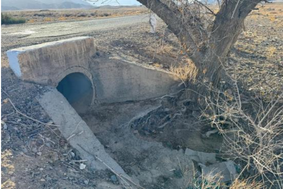
Photo 8. Condition of head/wing of drainage structures at outlet.
