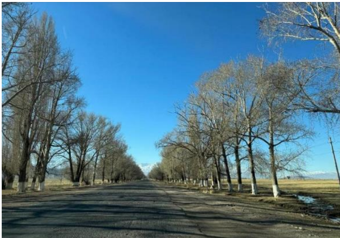
Photo 19. Route of Tendik-Roundabout road section.
