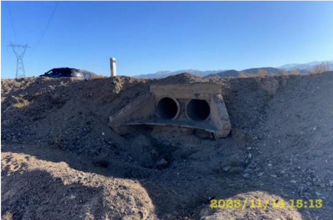
Photo 7. Condition of head/wing of drainage structures at outlet.
