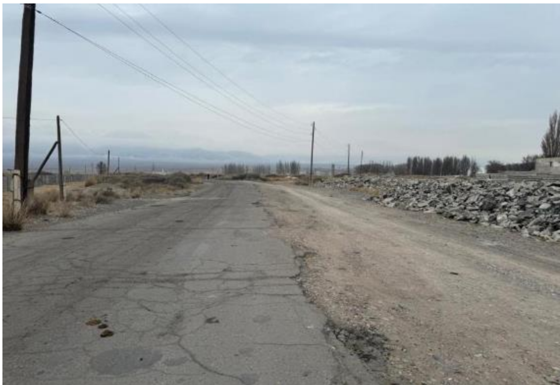
Photo 13. Beginning of street - adjacent to Balykchy-Kochkor road at chainage 1+725 LHS
