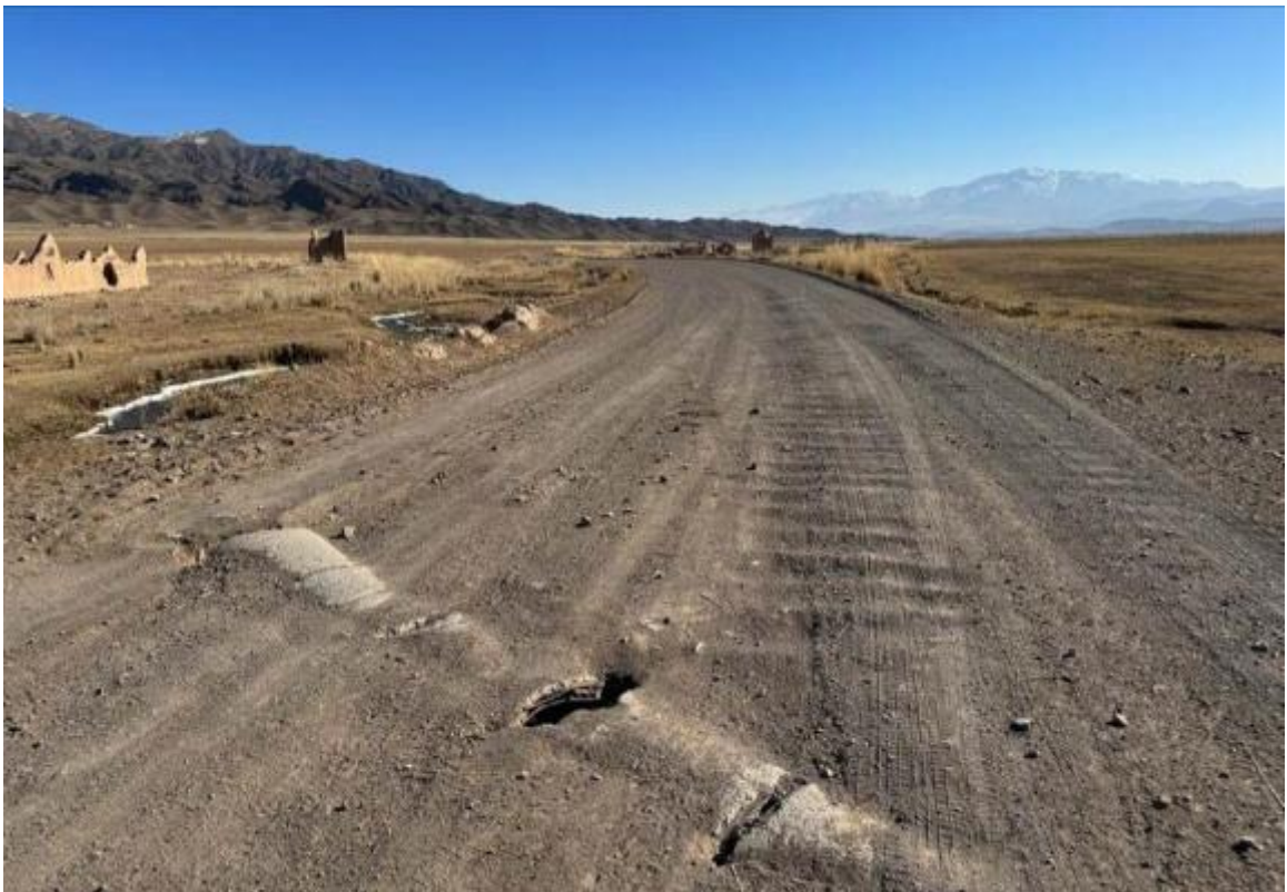
Photo 30. " Condition of water pipe.
