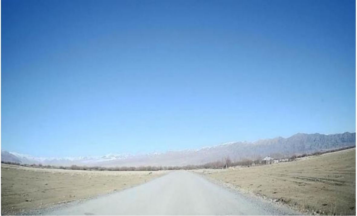
Photo 40. Beginning of section of Communism-Ortok road.
