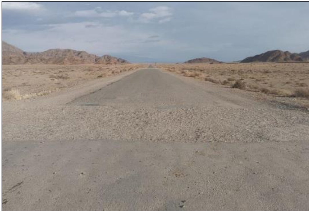
Photo 3. Road surface - old asphalt pavement.
